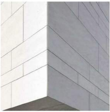
OFF WHITE EXPRESSED JOINTED PANEL CLADDING FC-02
